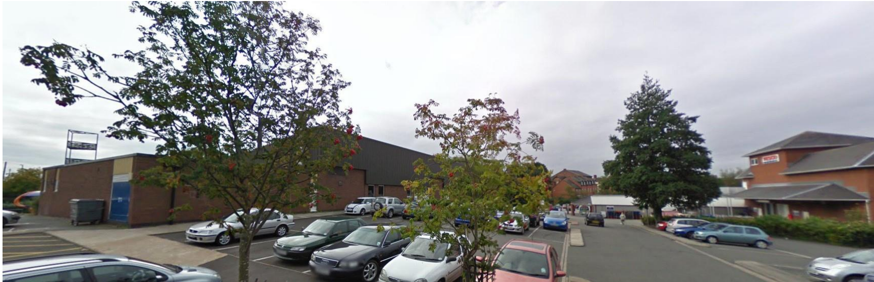
Showing existing swimming pool viewed from the north (view 2)
